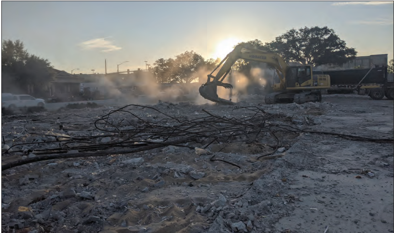
A. View Northeast of the Greyhound Bus Station Demolition
