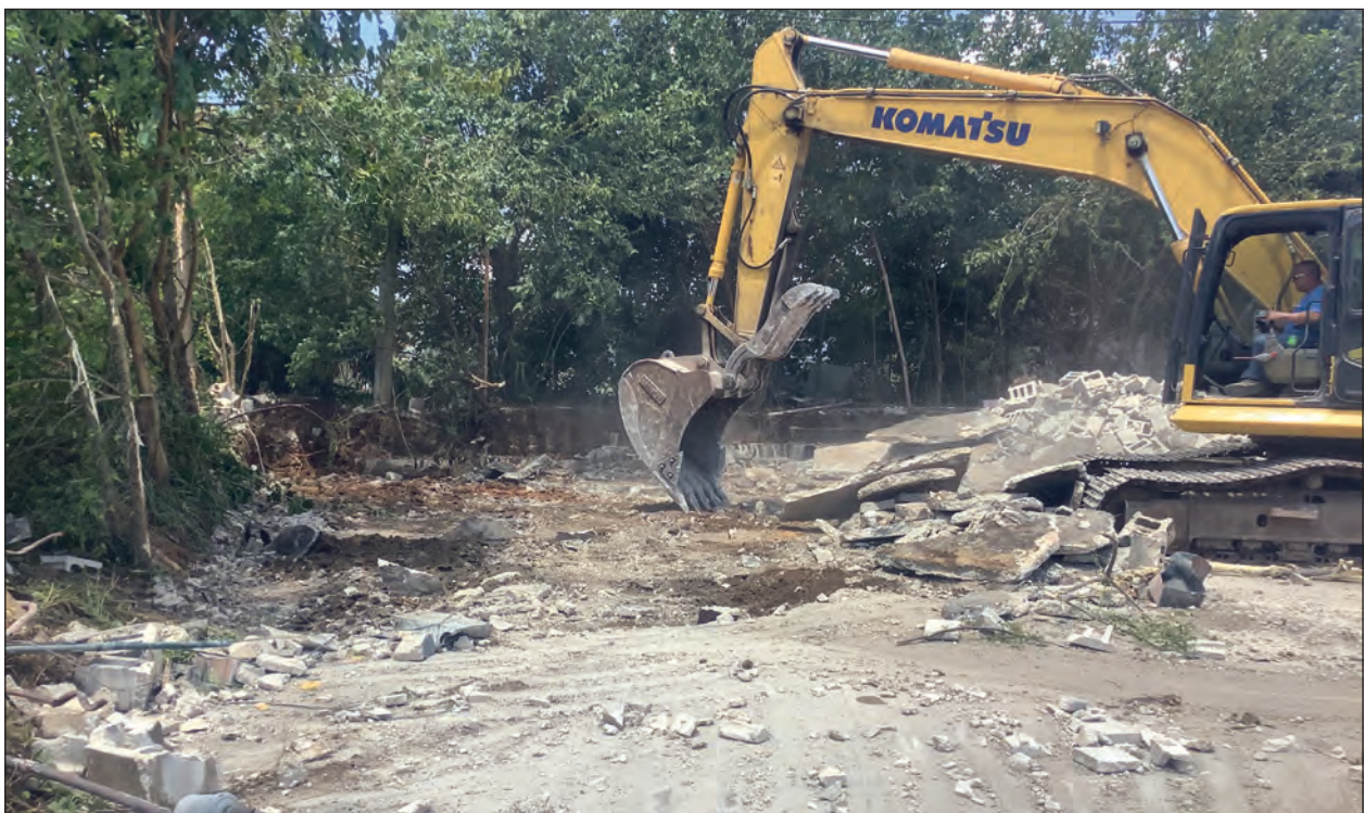
B. View East of the Red Fox Club Demolition
