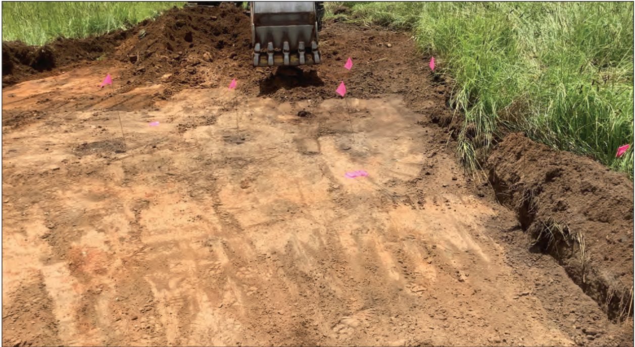
A. View South of Mechanical Stripping of Stripped Area B
